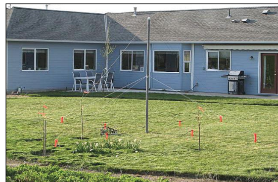
Figure 16 — Completed four element shared apex loop array utilizing two orthogonally positioned arrays identical to those described in this article.
