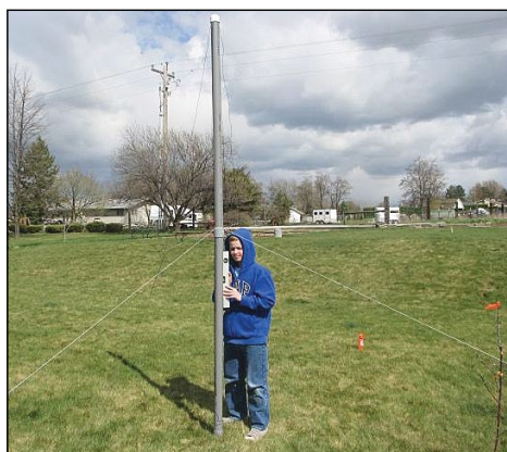
Figure 8 — Partially constructed array during mast alignment.
